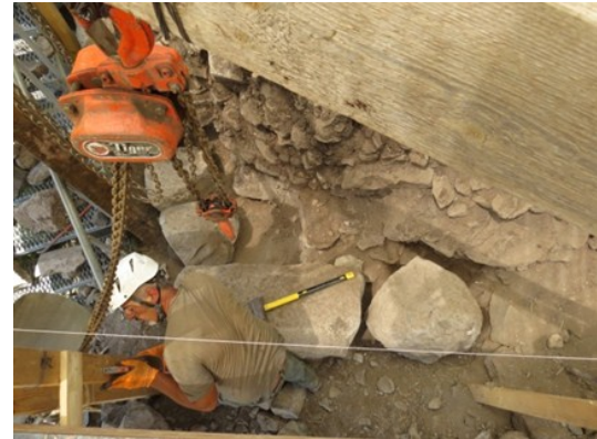
Fig. 3. Dismantling the wall.
