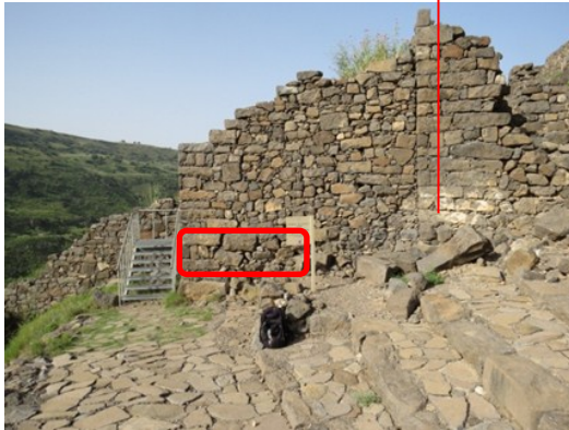
Fig. 2. The wall before the beginning of work, the area that swelled is marked in red.
